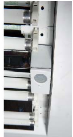
Close-up of Integral Occupancy Sensor in 6 Light Only
